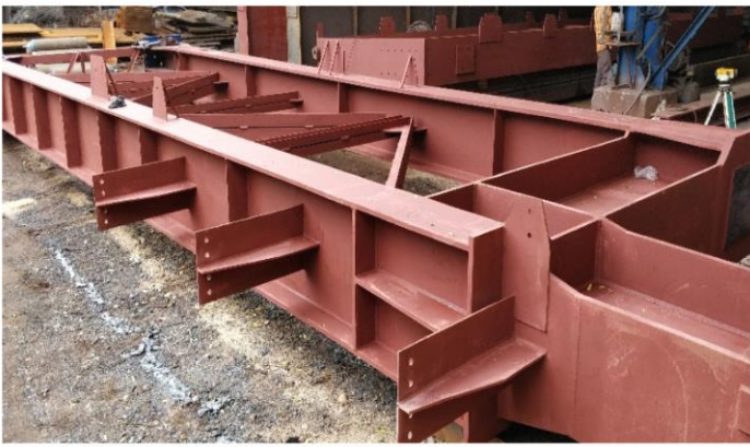
Fabricated Column for New HSM SAIL-RSP
